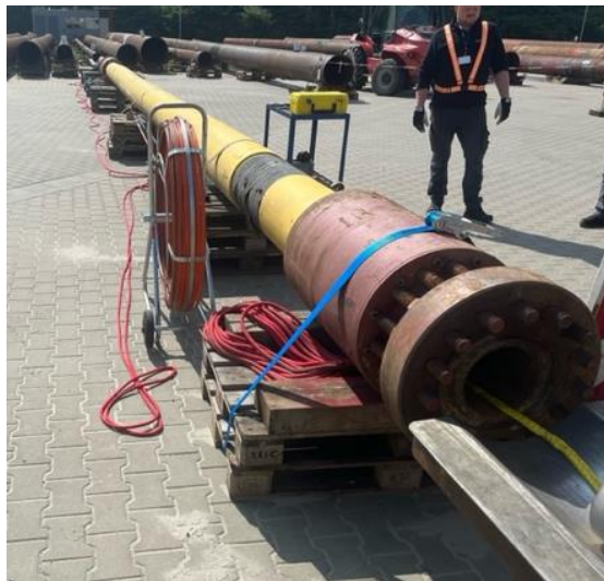
Figure 7: View along the installed flexible (yellow Dyneema® rope ready for pull)
